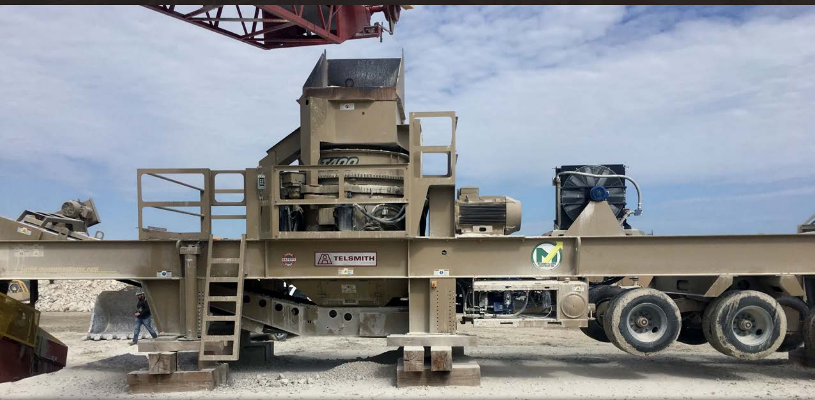
TERTIARY DOLOMITE CRUSHING
